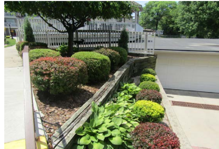
landscape and retaining wall
