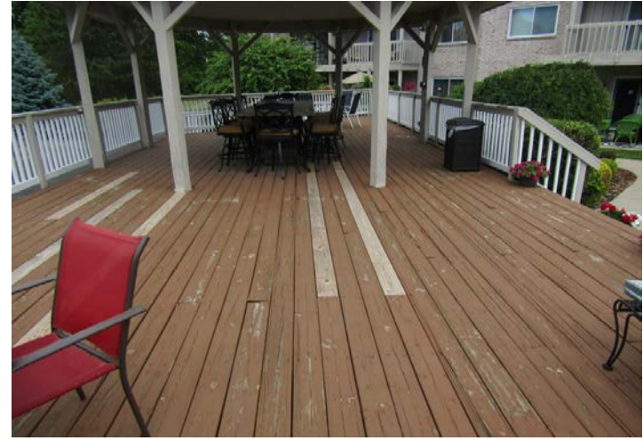
deck with wood frames, wood deck boards and wood railings
