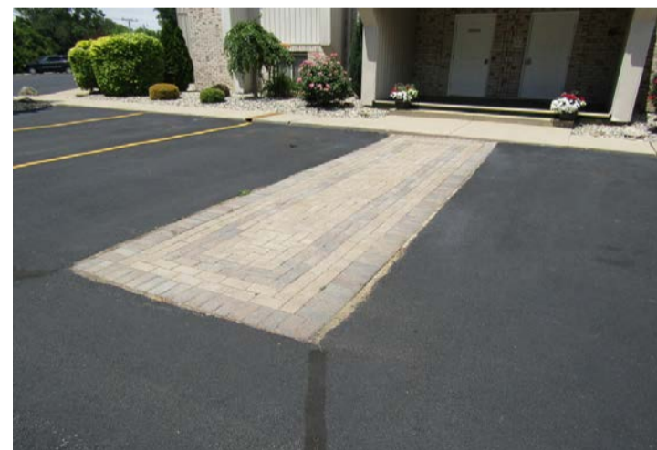
pavers at D entrance
