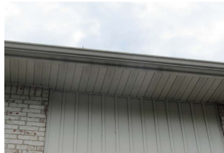
soffit and fascia
