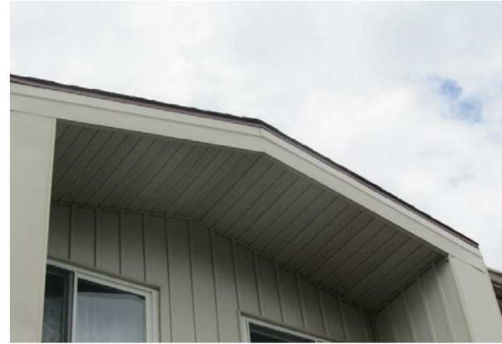
aluminum soffits and fascia
