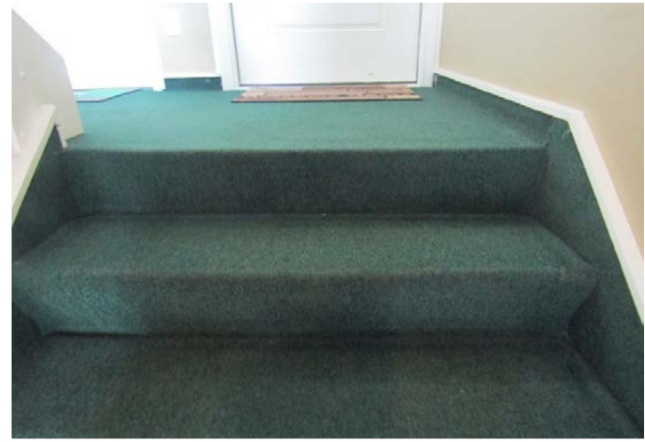
broadloom loop pile carpet typical of the stairs
