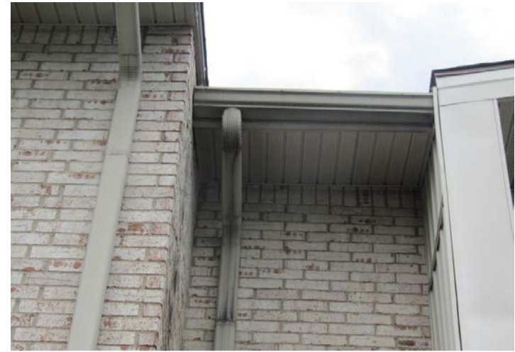
aluminum gutters and downspouts
