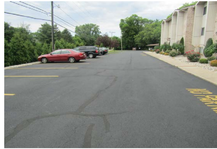
asphalt pavement at parking areas
