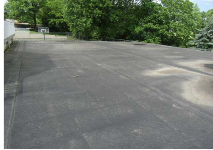
EPDM roof overview
