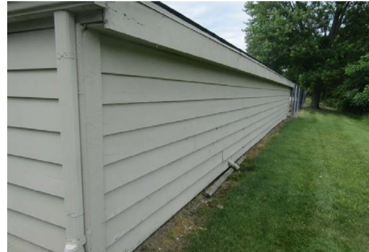
wood siding at garage
