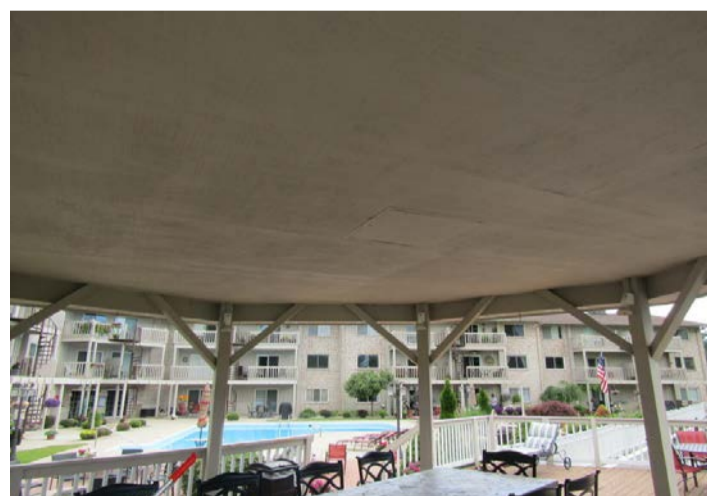
underside of gazebo
