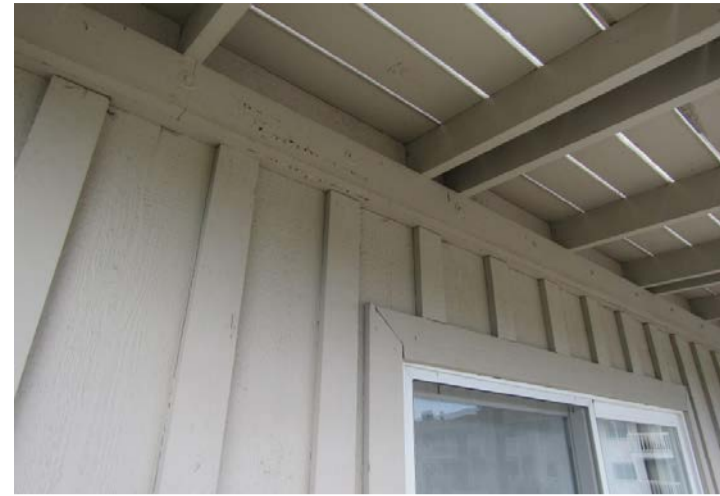
wood siding with board and batten profile
