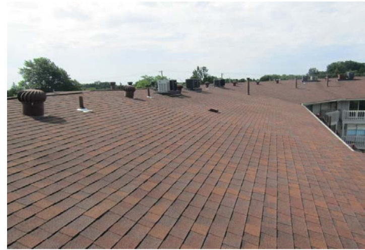
roof with asphalt shingles
