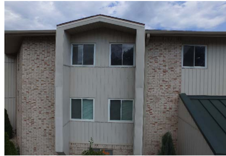
vinyl siding with ribbed profile
