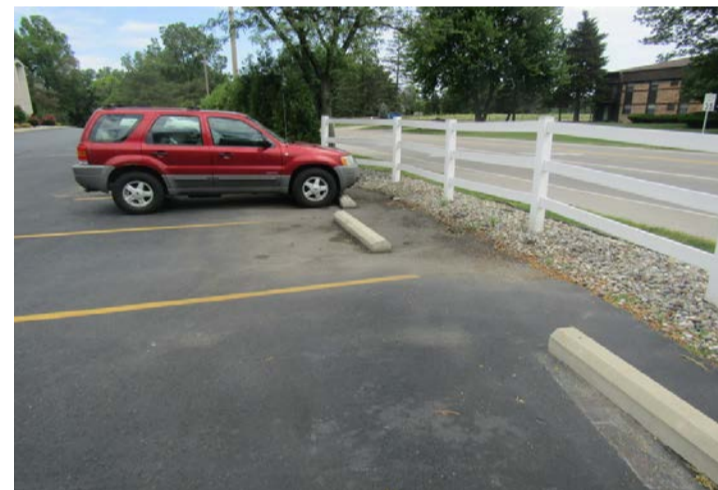
evidence of standing water - consider a French drain at this location
