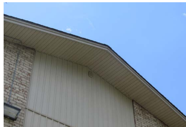
soffit and fascia
