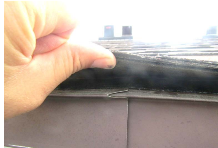
self adhering underlayment at gutter edge
