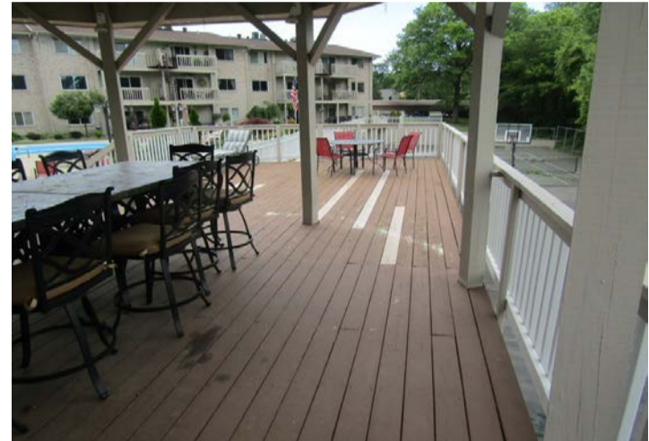
replaced deck boards
