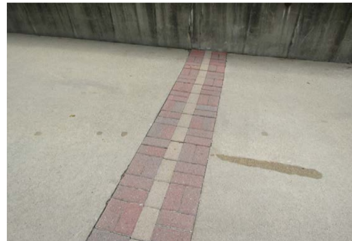
pavers at driveway
