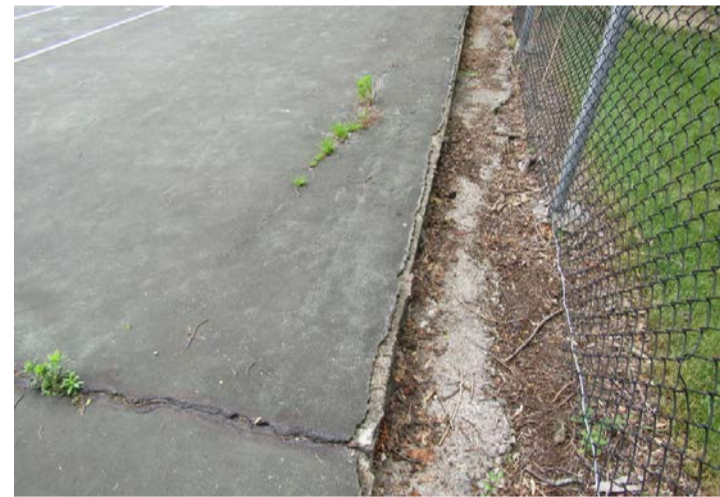
asphalt atop concrete slab
