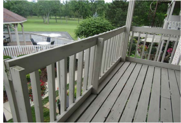
balconies with wood frames, wood deck boards and wood railings
