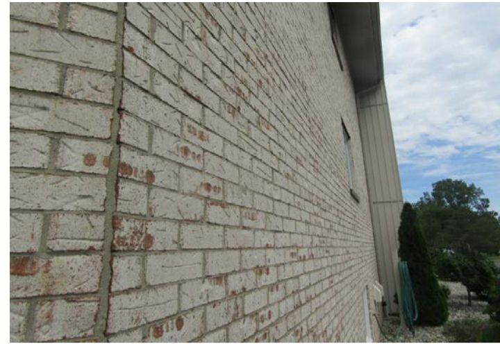
masonry facade with 3 by 10 inch masonry units and running bond pattern
